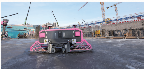
China Railway Construction Engineering Group Guangzhou Baiyun Station Project
